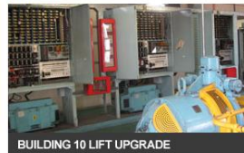
BUILDING 10 LIFT UPGRADE
