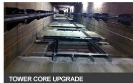
TOWER CORE UPGRADE
