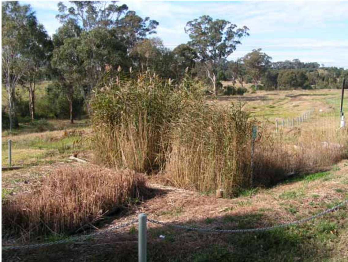
Reed beds for water filtration
